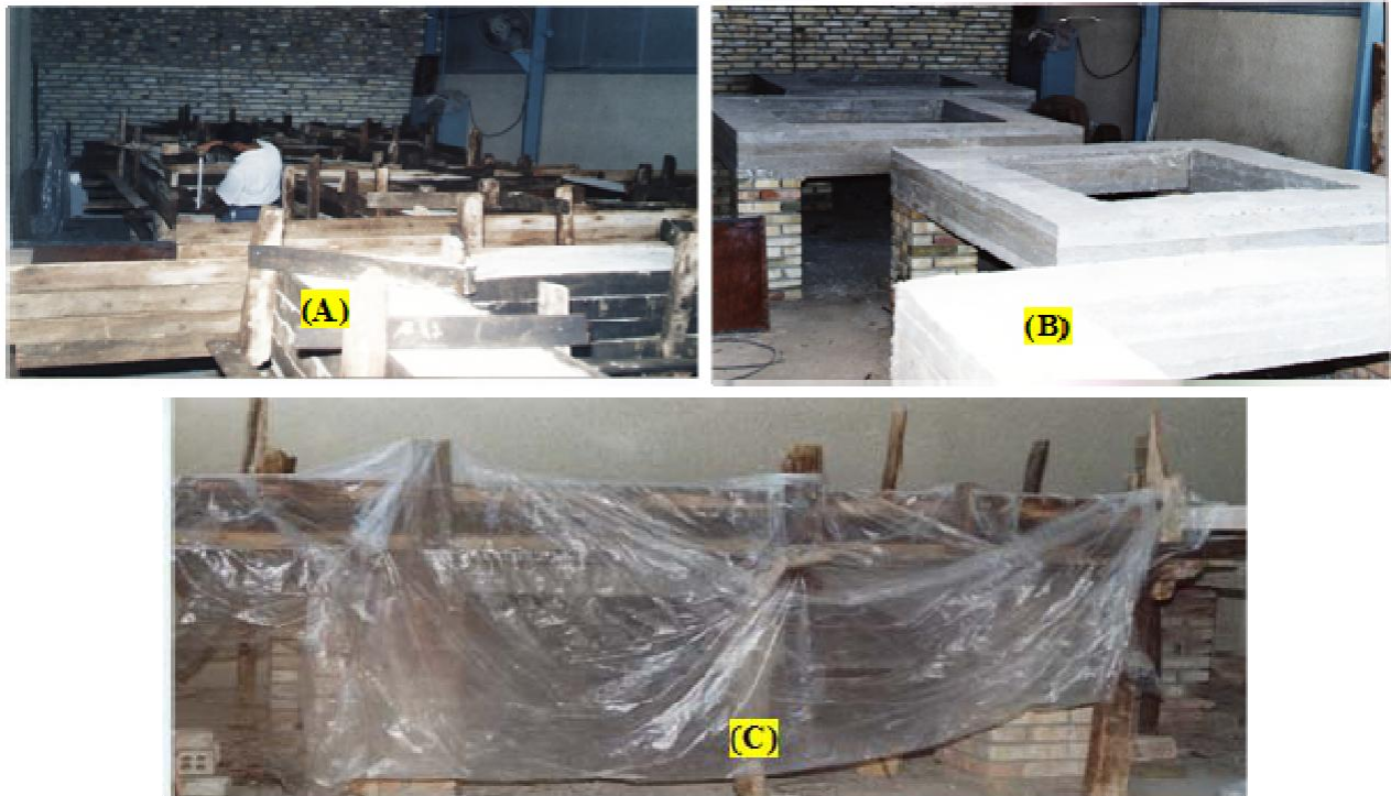
Figure 2. (A) The wood formwork of the rigid beams; (B) The rigid beams after lifting of the wood formwork; (C) Curing of Rigidbeam with the wetted hessian and polythene sheets.
